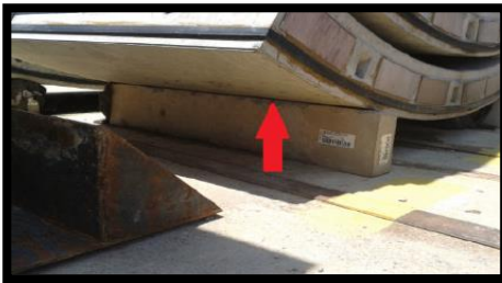
Figure 2.2.2: Precast panel stacked by concrete support. Source: [7].
