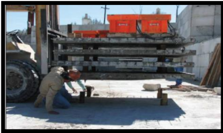
Figure 2.2.1: Precast panel lifted by forklift and stacked by timber. Source: [11].
